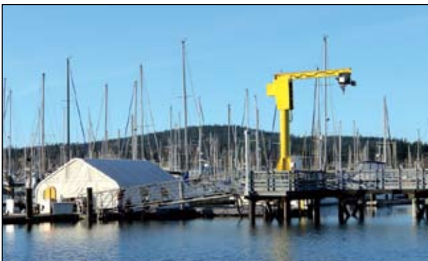
New small craft hoist at Cap Sante Boat Haven.
