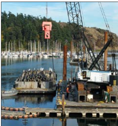
Old creosote pilings were removed last year.
