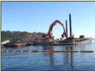
Fidalgo Bay dredging, Cap Sante in the background. A great quantity of wood debris and pilings have been dredged.
