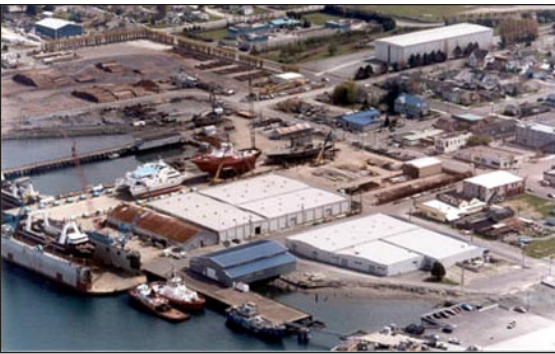
DCI with synchrolift, drydock and upland facility.
